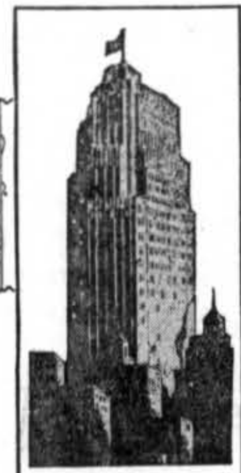
TELEPHONE BUILDING PAINTED AND LACQUERED - BY A. QUANDT & SONS
