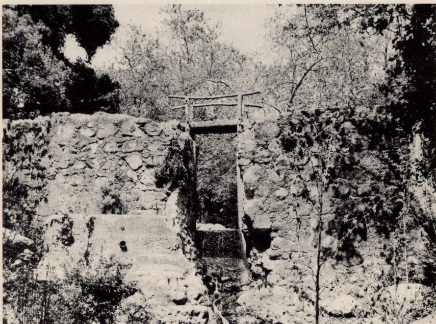
FIGURE 245. ". . . . A DAM OF ROUGH STONE AND MORTAR . . . ." The Santa Barbara Mission dam. Photo by courtesy of Anderson Photo Service, Santa Barbara.
