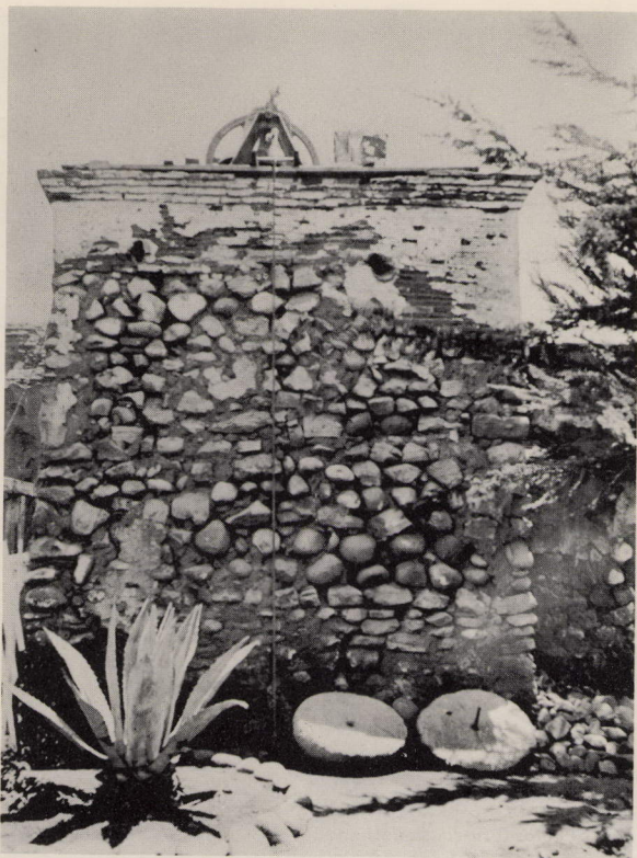
FIGURE 257. BRICK, PEBBLES, AND STONE IN THE BELL TOWER AT MISSION SAN DIEGO DE ALCALÁ, 1905. Photo from the collection of the California Historical Society.
