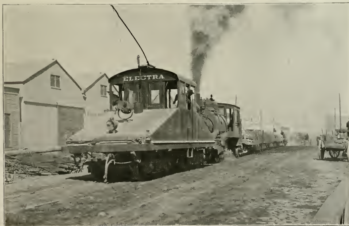
ELECTRIC AND STEAM POWER EMPLOYED TO REMOVE DEBRIS BY RAIL
