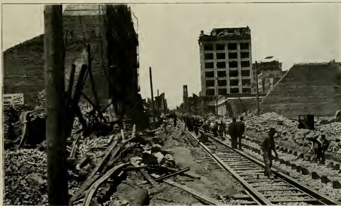
REPLACING THE SUTTER STREET CABLE WITH AN ELECTRIC LINE IMMEDIATELY AFTER THE FIRE View west from Market Street
