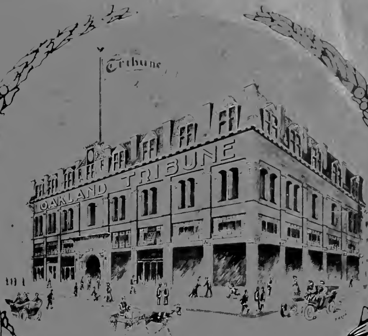
NEW TRIBUNE BLDG COR 8TH & FRANKLIN.
