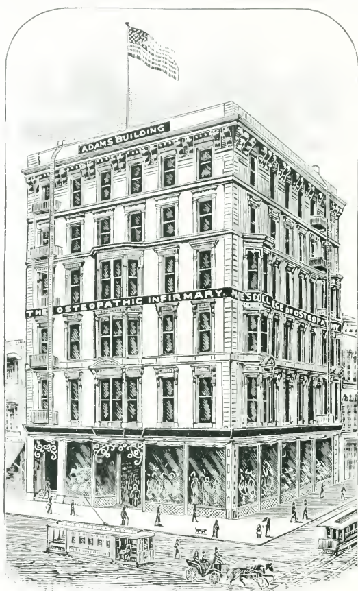
ADAMS BUILDING, 206 Kearny St., Cor. Sutter
