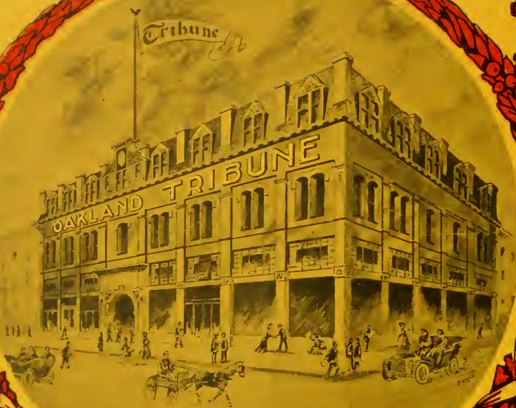
NEW TRIBUNE BLDG COR 8TH & FRANKLIN.
