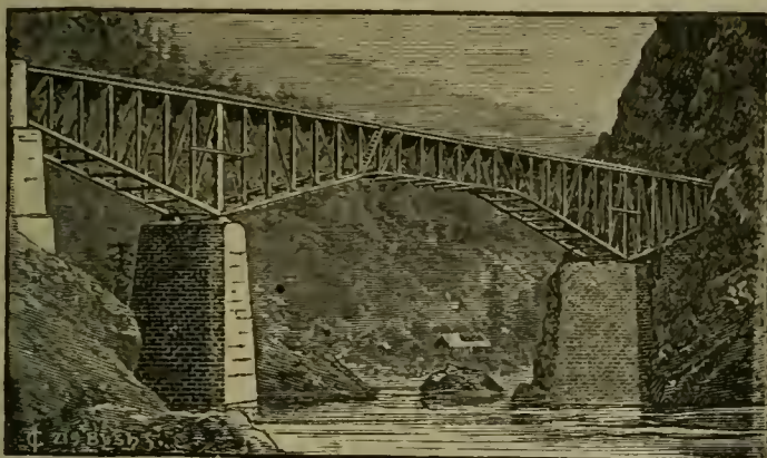
Centre Span 315 feet. Erected in 1884 by S. F. Bridge Co. in 73 days.
